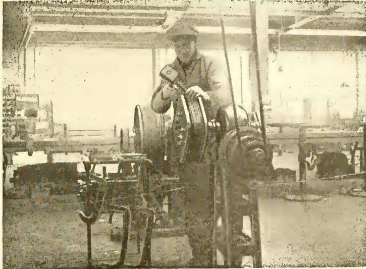
On the job at Portland, Ore.
