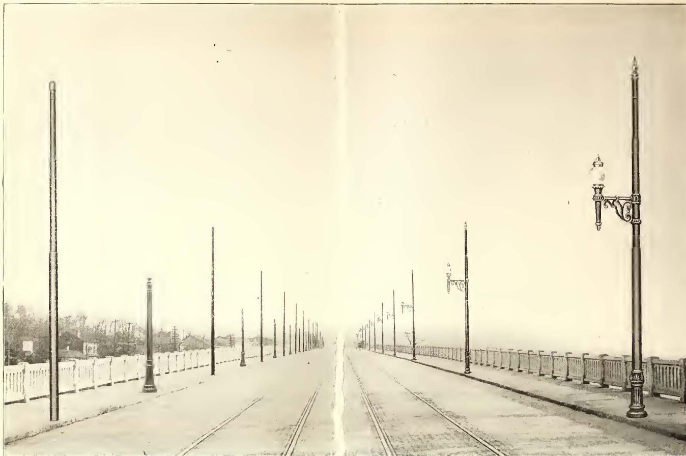
Two Sets of Poles Double Expense.
