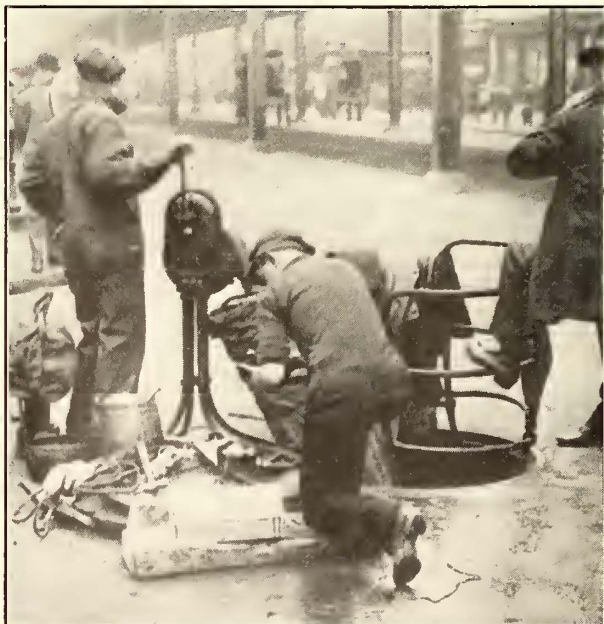
FREEING MANHOLES OF GAS—HAND-DRIVEN BLOWER AT WORK
