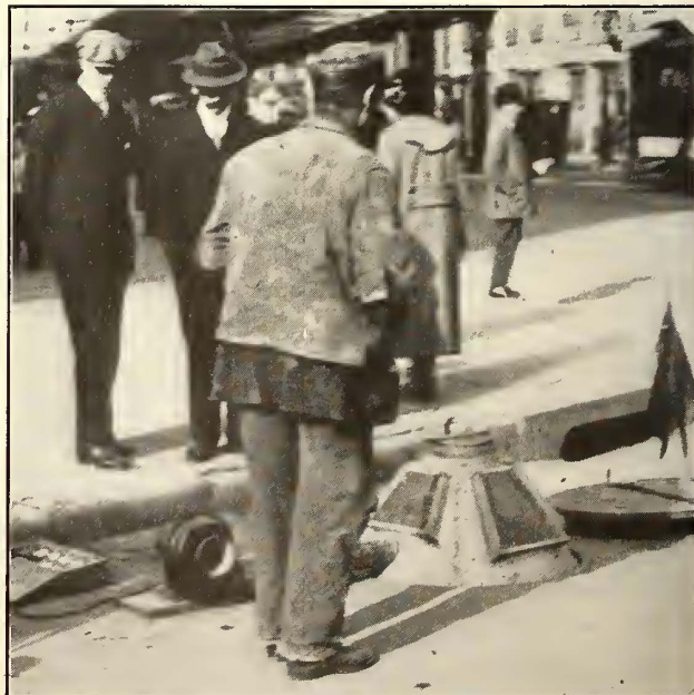
FREEING MANHOLES OF GAS—MANHOLE HOOD FOR USE IN PUTTING MANHOLE UNDER AIR PRESSURE
