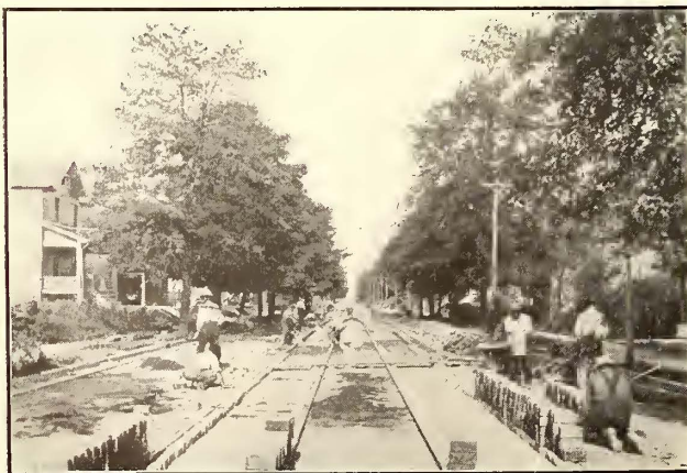
TRACK REHABILITATION IN SPRINGFIELD—PAVING TRACK IN WEST PLEASANT STREET, SPECIAL-WORK LAYOUT WITH STEEL TIES
