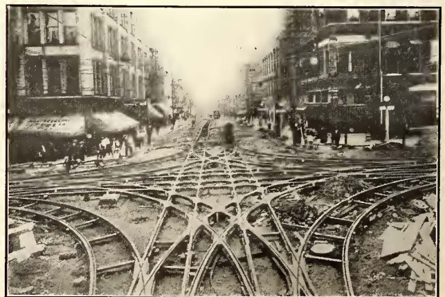
TRACK REHABILITATION IN SPRINGFIELD—PAVING TRACK IN WEST PLEASANT STREET, SPECIAL-WORK LAYOUT WITH STEEL TIES
