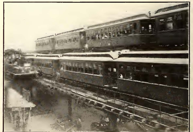
MANHATTAN ELEVATED THIRD TRACKING—RAISED THIRD TRACK PRIOR TO ERECTION OF EXPRESS STATION
