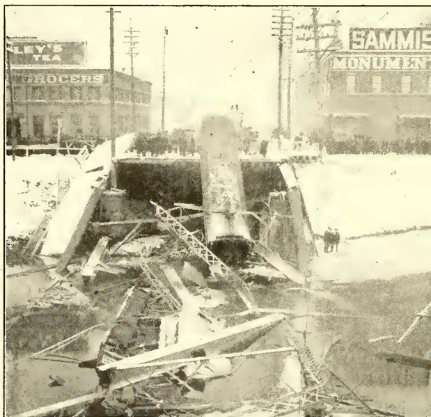
SPOKANE BRIDGE FAILURE—VIEW SHOWING CAR CAUGHT ON EDGE OF BRIDGE AND SEATS OF SUBMERGED CAR IN WHICH FATALITIES OCCURRED
