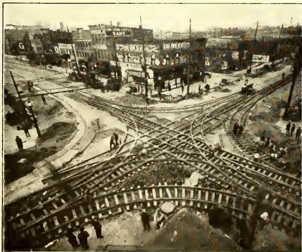
COMPLICATED SPECIAL-WORK LAYOUT AT BUSY STREET INTERSECTION IN AKRON
