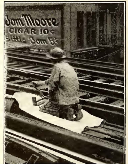
SAFETY ON THE CHICAGO ELEVATED—PROTECTION IN CABLE SPlicing; PROTECTION IN TRACK WORK; CANVAS PROTECTION IN THIRD-RAIL WORK
