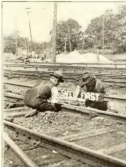
SAFETY ON THE CHICAGO ELEVATED—PROTECTION IN CABLE SPlicing; PROTECTION IN TRACK WORK; CANVAS PROTECTION IN THIRD-RAIL WORK
