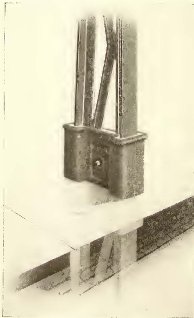
CAST-IRON SLEEVE TO PREVENT CORROSION OF STEEL POLES
