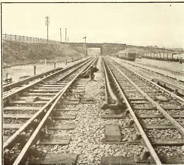
LANCASHIRE & YORKSHIRE ELECTRIFICATION—VIEW SHOWING FOURTH-RAIL RETURN; VESTIBULE DOORS ON CARS
