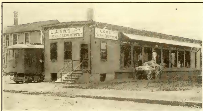
BUILDING UP A FREIGHT BUSINESS—FIRST FREIGHT SHED IN LEWISTON, ME., L. A. & W. ST. RY., BUILT JUNE, 1915
