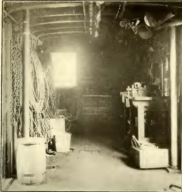
OVERHEAD CONSTRUCTION—INTERIOR OF CONNECTICUT COMPANY TOWER CAR; BENCH END
