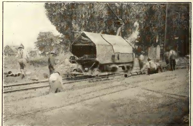
CLEVELAND TRACK COSTS—SURFACING JOINTS WITH GRINDER
