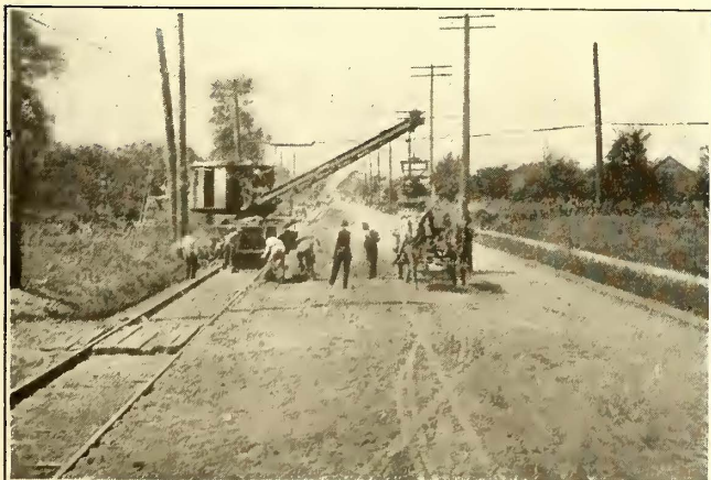
CLEVELAND TRACK COSTS—CLAMSHELL DERRICK CLEANING UP WORK
