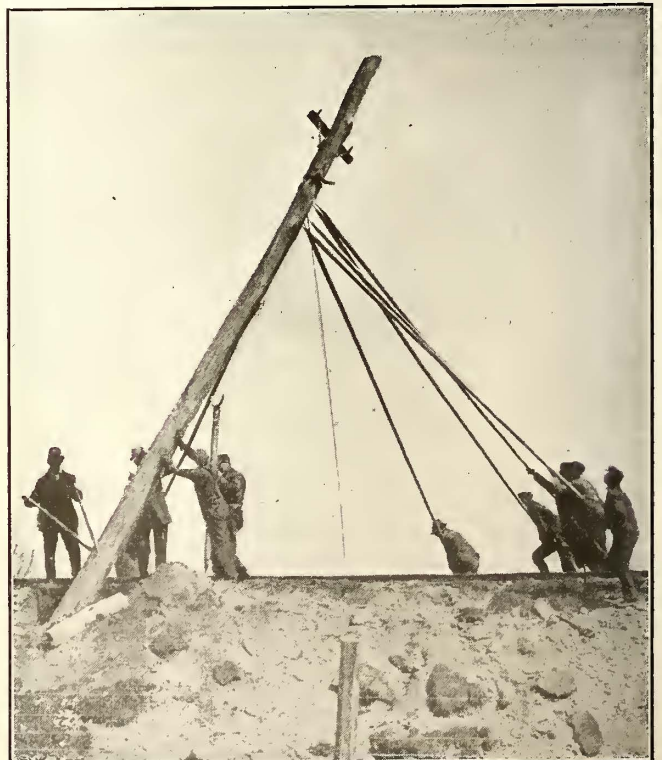
OVERHEAD CONSTRUCTION—HOME-MADE YET VERY EFFICIENT POLE SETTER; NOTE ANCHOR GRIP ON RAIL OPPOSITE POLE BETWEEN WHEELS. POLE ERECTION BY HAND
