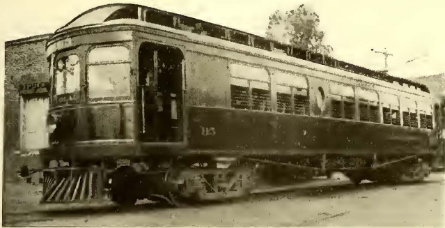
VIEW OF COMPLETED CAR WITH SHEET STEEL SIDING
