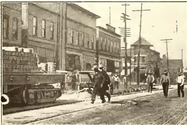
CLEVELAND TRACK COSTS—PAVEMENT ROOTER IN OPERATION
