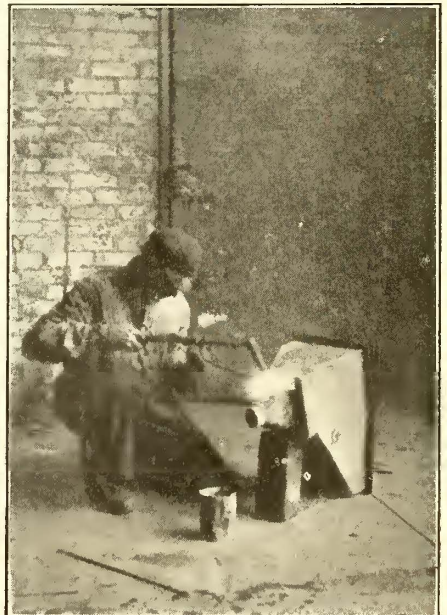
OXY-ACETYLENE REPAIRS—WELDING BROKEN SAND BOX IN FIFTEEN MINUTES
