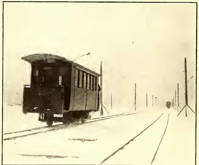
TEMPORARY TRACK OVER THE NEVA RIVER
