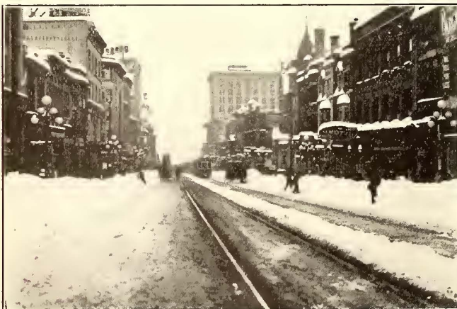
VIEW ON GRANVILLE STREET, LOOKING NORTH FROM GEORGIA STREET
