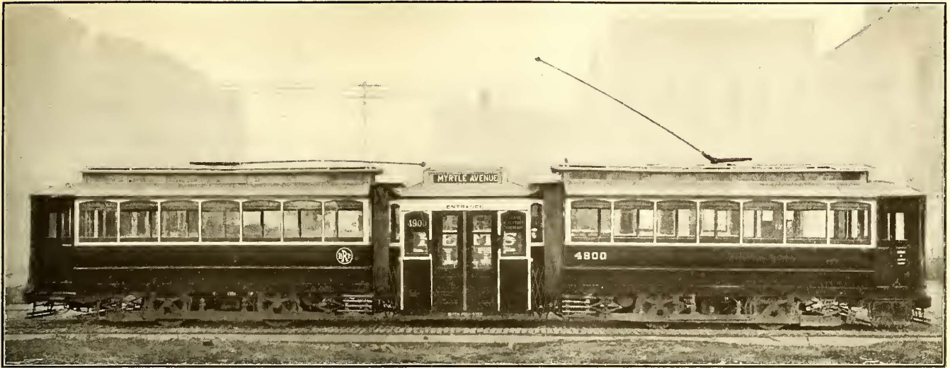
BROOKLYN ARTICULATED CAR—SIDE VIEW OF NEW CAR, 62 FEET, 10 INCHES OVER ALL
