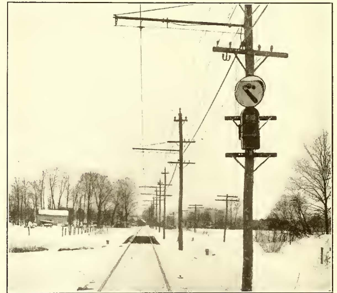
TYPICAL HIGH-SPEED INTERURBAN SIGNAL ON JAMESTOWN, WESTFIELD & NORTHERN RAILROAD
