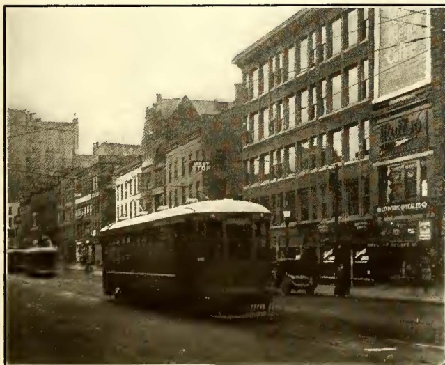
ELECTRIC TRACK SWITCH AT CONGESTED CORNER IN ROCHESTER
