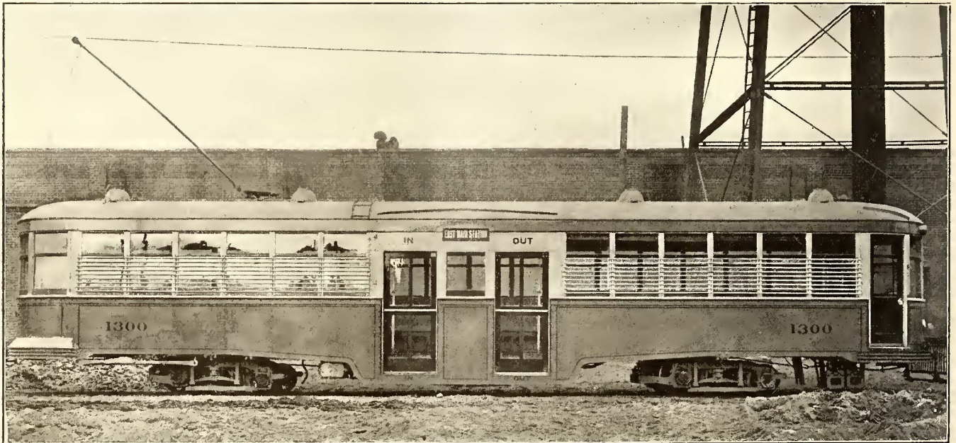
ROCHESTER CAR—GENERAL VIEW OF CAR SHOWING ARRANGEMENT OF ENTRANCE AND EXITS DOORS
