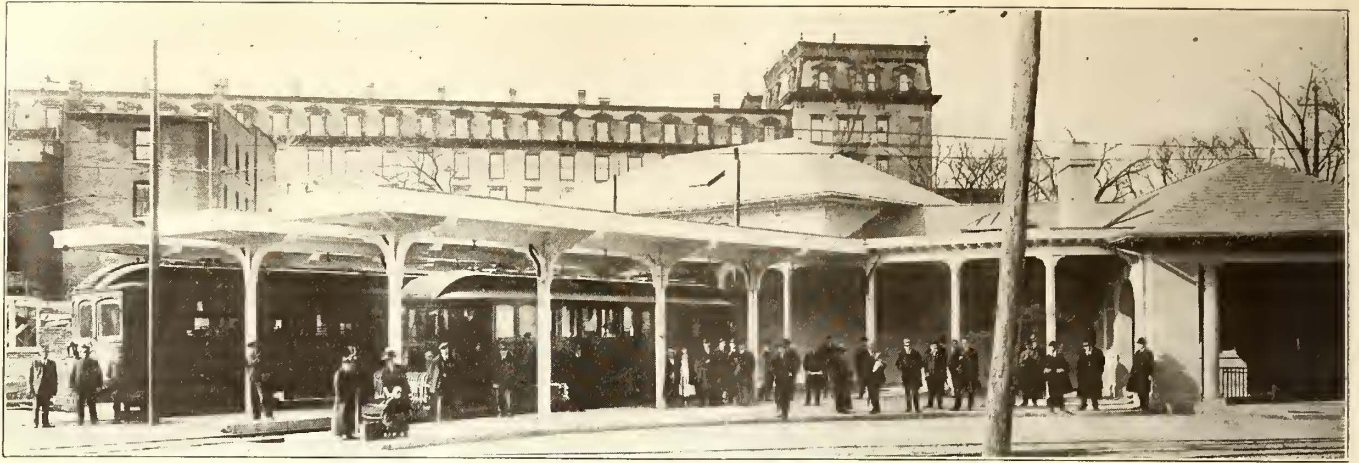
VIEW OF TERMINAL, SHOWING CARS, PLATFORMS, AND TRAIN SHEDS
