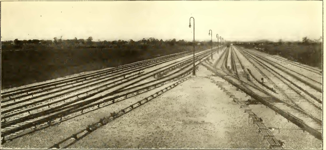
DETROIT RIVER TUNNEL OPERATION—ELECTRIC PICK-UP YARD IN WINDSOR
