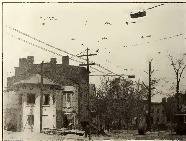
P. S. TERMINAL SIGNALING—MULBERRY STREET TOWER
