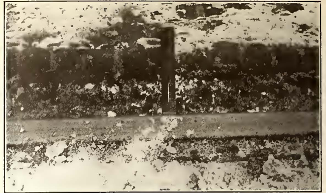
MORE ILLUSTRATIONS OF DAMAGE TO BRICK PAVEMENT. IN ONE CASE REMOVAL OF BRICK WAS NECESSARY. IN THE OTHER THE HEAVE WAS 5 IN.
