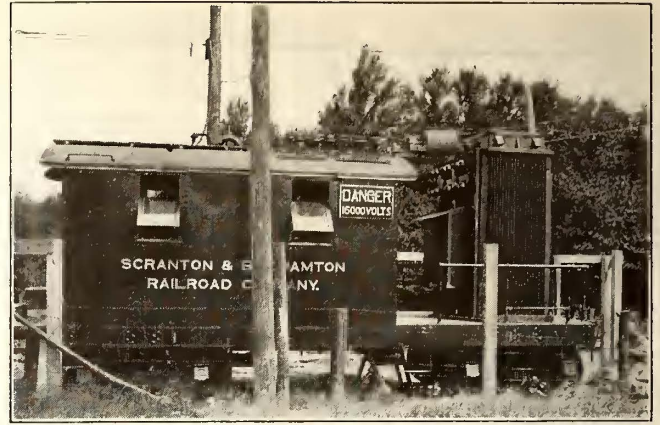
SCRANTON &amp; BINGHAMTON TRAFFIC—PORTABLE SUBSTATION
