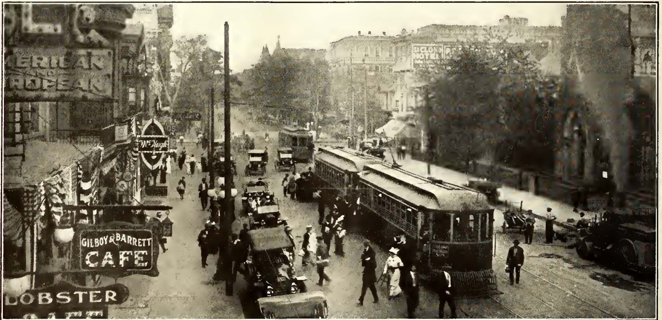
SCRANTON & BINGHAMTON TRAFFIC—PASSENGER TERMINAL AT SCRANTON
