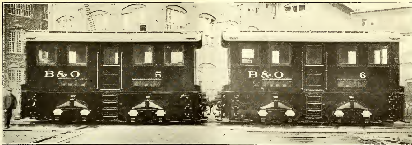
B. & O. ELECTRIFICATION—TWO 80-TON LOCOMOTIVES OF 1903 TYPE
