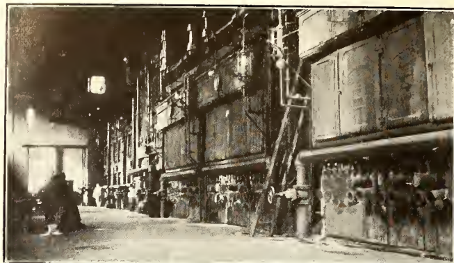
BANK OF BOILERS IN ELYRIA POWER STATION EQUIPPED TO BURN GAS FOR FUEL; INTERIOR OF GAS REGULATOR AND METER HOUSE
