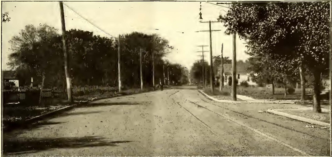
Rockingham Road, Davenport, Iowa. Brick pavement filled with Barrett's Paving Pitch.
