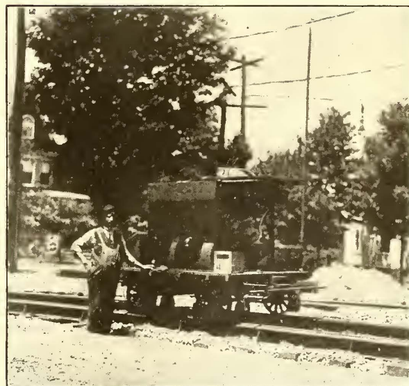
The Public Service Railway Co. of New Jersey is using a two-tool Imperial Tamping Outfit for extension work on the Central Ave. line, East Orange, N. J. The portable compressor which operates the tampers is electrically driven from the trolley line. N. B. The Ingersoll-Rand Company also builds gasoline driven compressors for conditions where electric current is unavailable.
