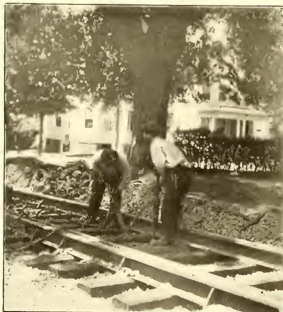
The Public Service Railway Co. of New Jersey is using a two-tool Imperial Tamping Outfit for extension work on the Central Ave. line, East Orange, N. J. The portable compressor which operates the tampers is electrically driven from the trolley line. N. B. The Ingersoll-Rand Company also builds gasoline driven compressors for conditions where electric current is unavailable.
