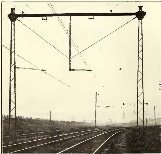
BRITISH FREIGHT ELECTRIFICATION—OVERHEAD CONSTRUCTION AT CURVE
