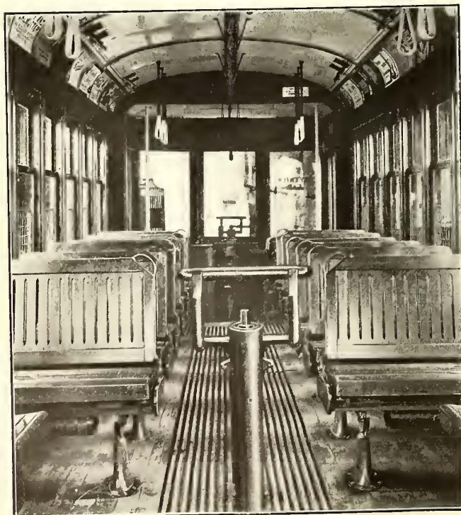
INTERIOR VIEW OF ALBANY CAR
