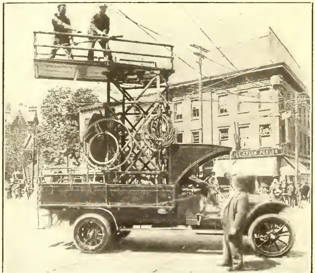
THIRD AVENUE LINE TRUCKS—TOWER TRUCK USED BY YONKERS RAILROAD
