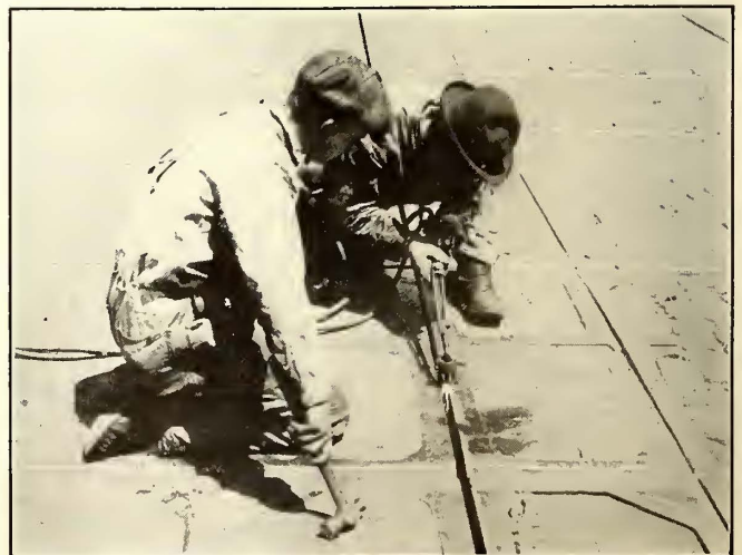
WIDENING CABLE SLOT IN SAN FRANCISCO WITH OXY-ACETYLENE FLAME
