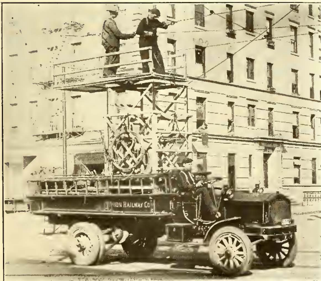
THIRD AVENUE LINE TRUCKS—3-TON TRUCK ON ORIGINAL PNEUMATIC TIRES
