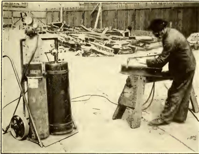
CUTTING RAILS IN IRREGULAR SHAPES WITH OXY-ACETYLENE FLAME
