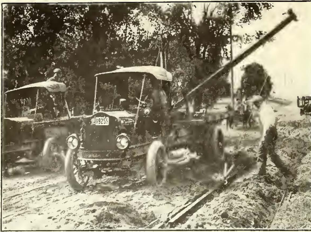
TEARING UP ABANDONED RAILWAY TRACK WITH DOUBLE-DRUM POWER WINCH AND BOOM; EMERGENCY LINE TRUCKS FULLY EQUIPPED
