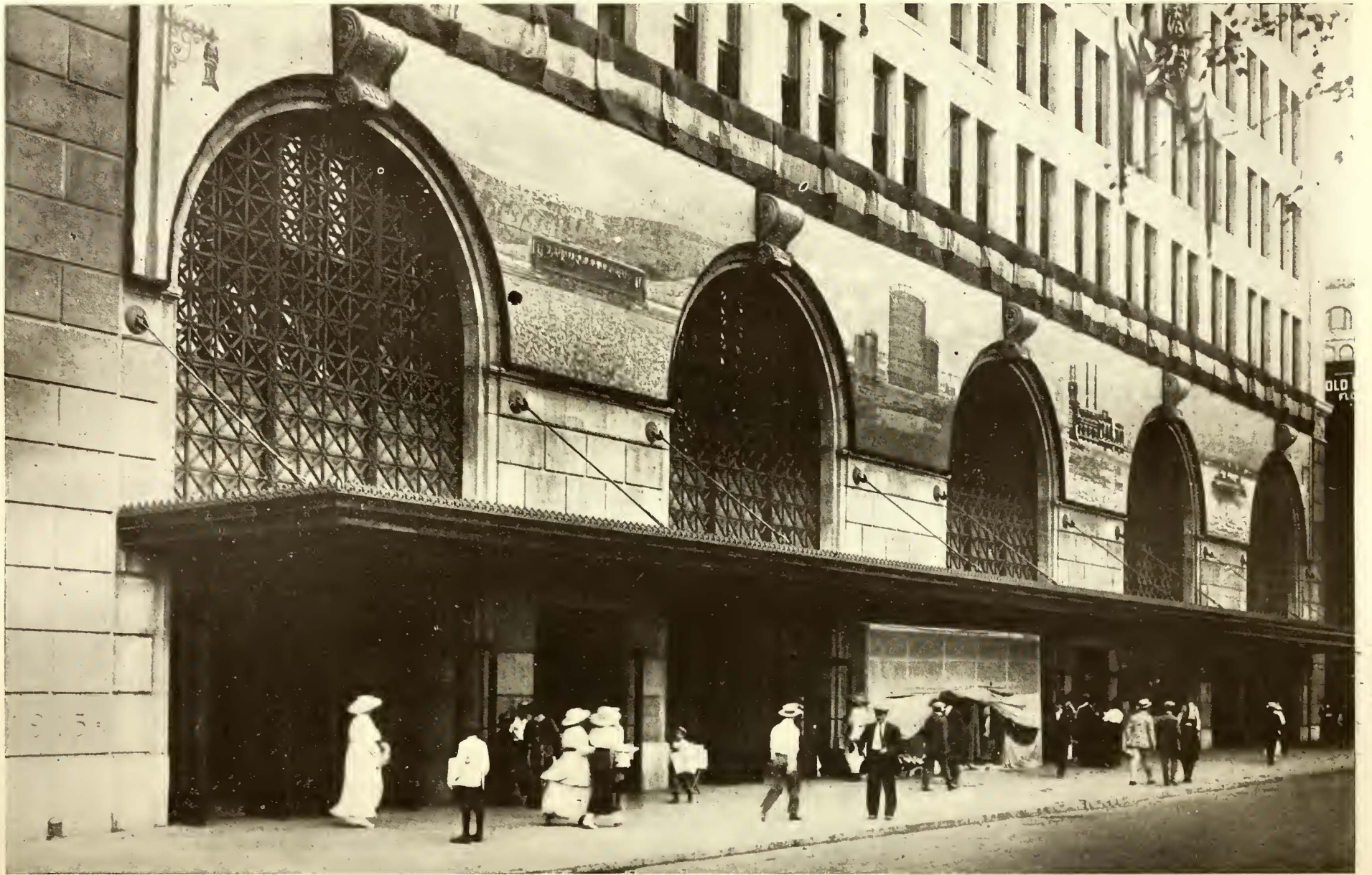
Façade of Public Service Terminal Building on Park Place, Newark, N. J. Paintings above marquee are in honor of Newark's 250th Anniversary Celebration
