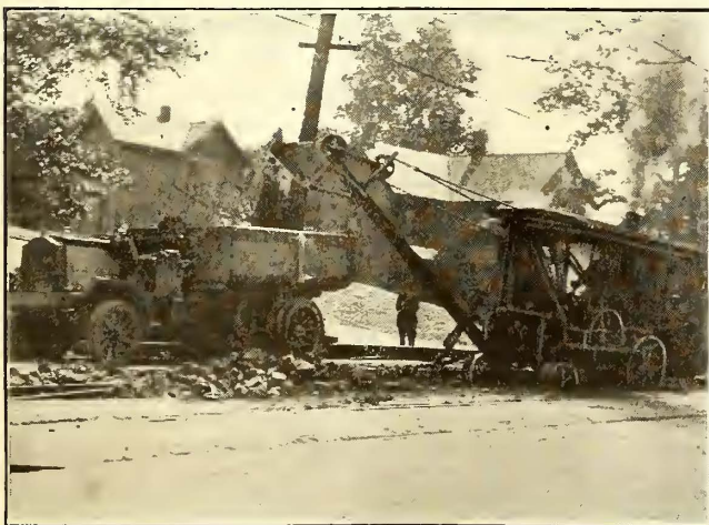
LIMITED CLEARANCE STEAM SHOVEL IN DUMPING POSITION
