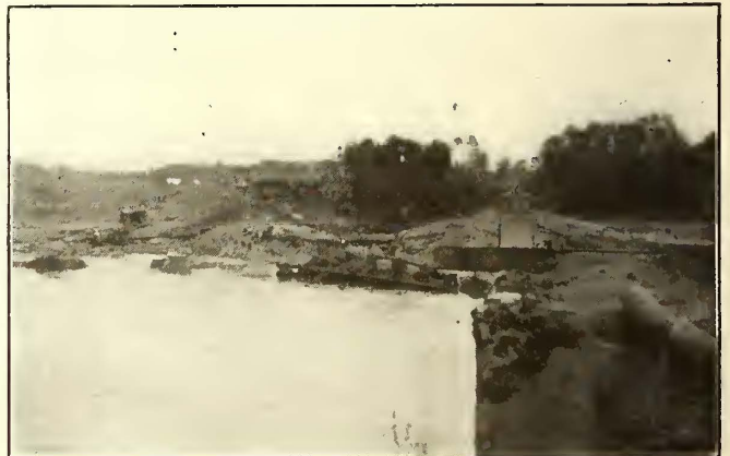
LOCATION NEAR MT. HOLLY (N. C.), SHOWING ALL THAT REMAINS OF THREE BRIDGES
