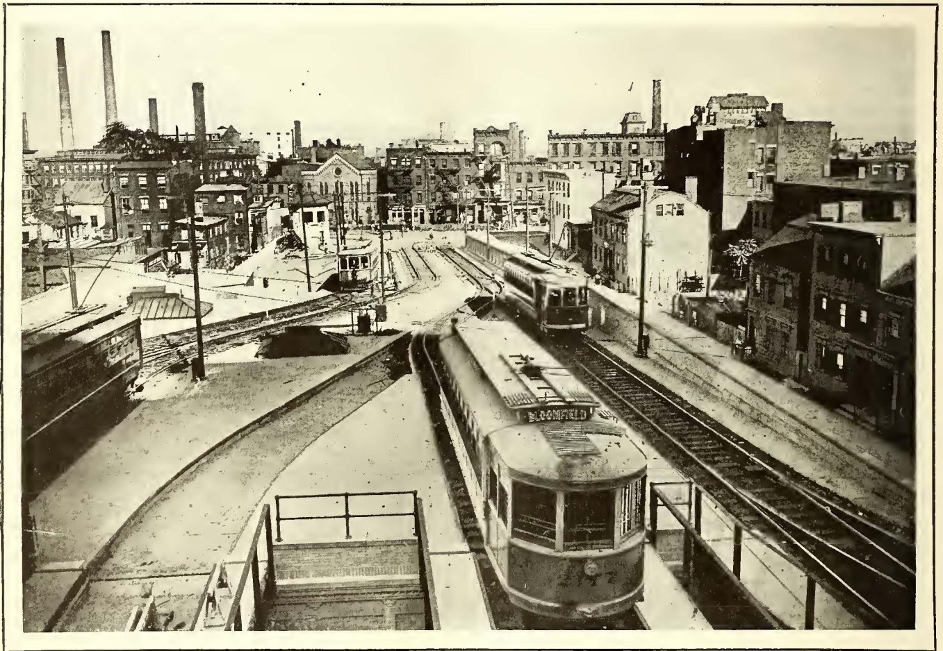
PUBLIC SERVICE RAILWAY REROUTING—VIEW FROM REAR OF TERMINAL ELEVATED FLOOR LOOKING TOWARD MULBERRY STREET
