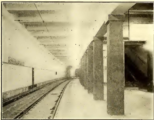
BOSTON STATION IMPROVEMENTS—SCOLLAY UNDER STATION ON EAST BOSTON TUNNEL EXTENSION
