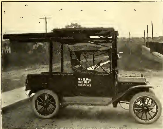
EMERGENCY LINE CAR—LADDER AND PLATFORM IN FOLDED POSITION
