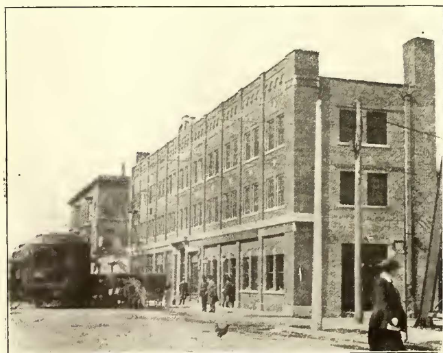
FORT DODGE LINE—VIEW OF NEW TERMINAL BUILDING AT FORT DODGE
