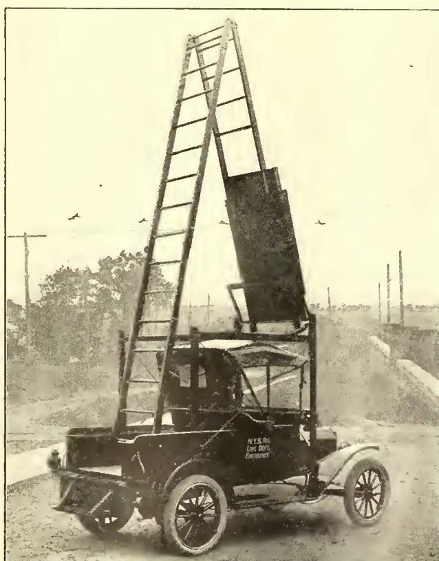
EMERGENCY LINE CAR—VIEW SHOWING LADDER IN RAISED POSITION
