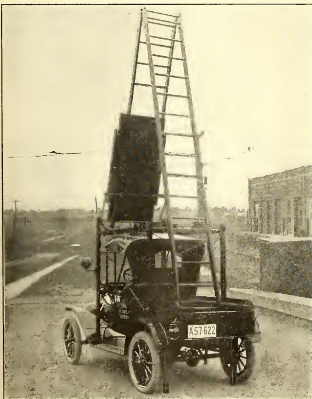
EMERGENCY LINE CAR—SHOWING SEARCHLIGHT, GONG, CLOSED TAILBOARD, AND LOWERED SPUDS
