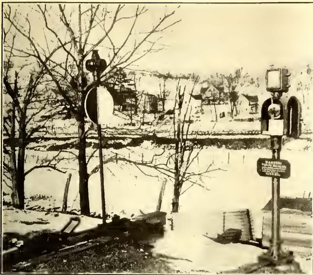
SCRANTON & BINGHAMTON SIGNALS—SWITCH INDICATOR AT OUTLYING PASSING SIDING
