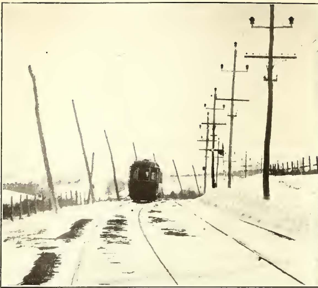
SCRANTON & BINGHAMTON SIGNALS—HOME SIGNAL WITH DIRECTION INDICATOR TWO POLES IN ADVANCE
