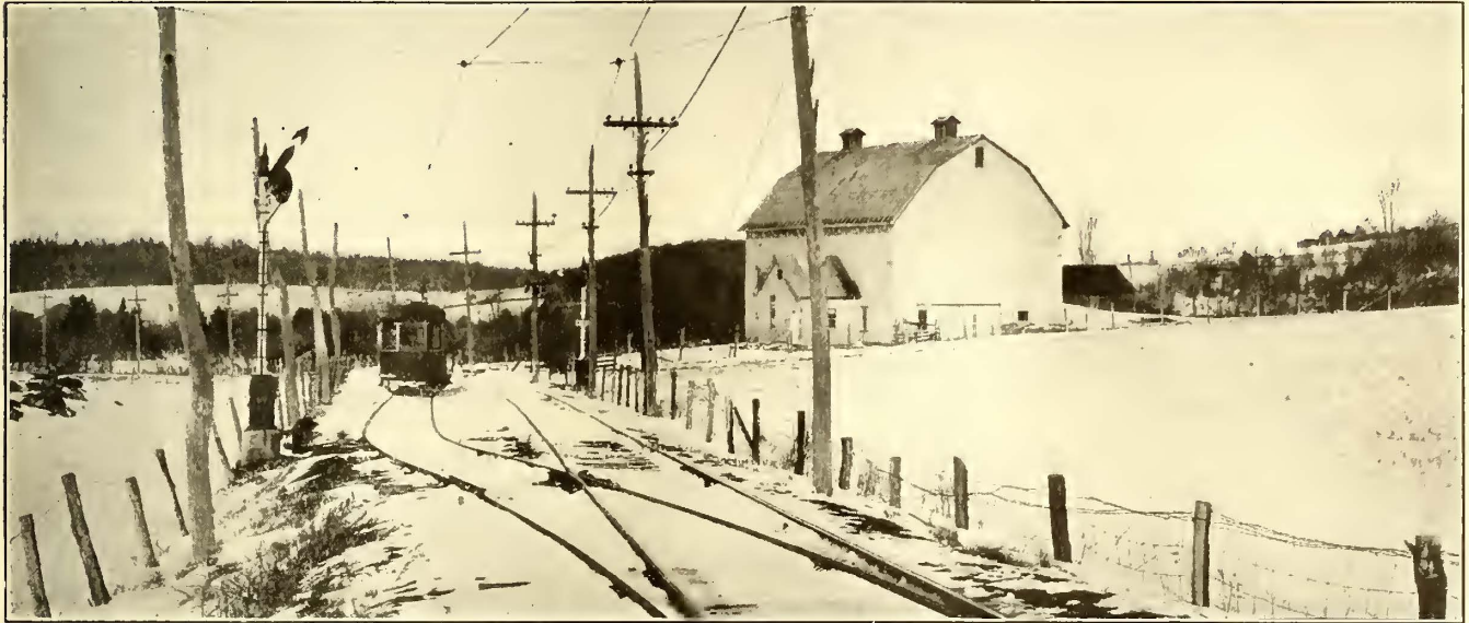
SCRANTON & BINGHAMTON SIGNALS—HOME SIGNAL AT PASSING SIDING
