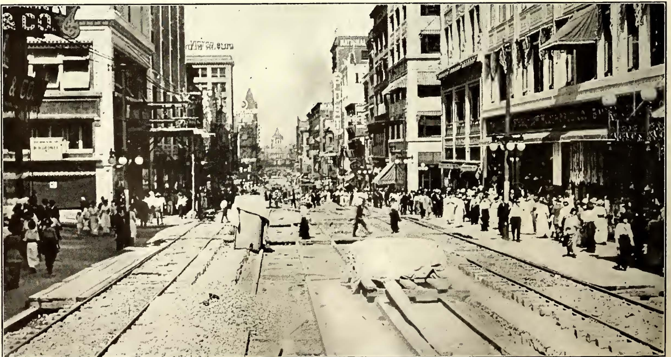
KANSAS CITY TRACK CONSTRUCTION—VIEW OF BUSINESS STREET ABANDONED FOR TRACK WORK
