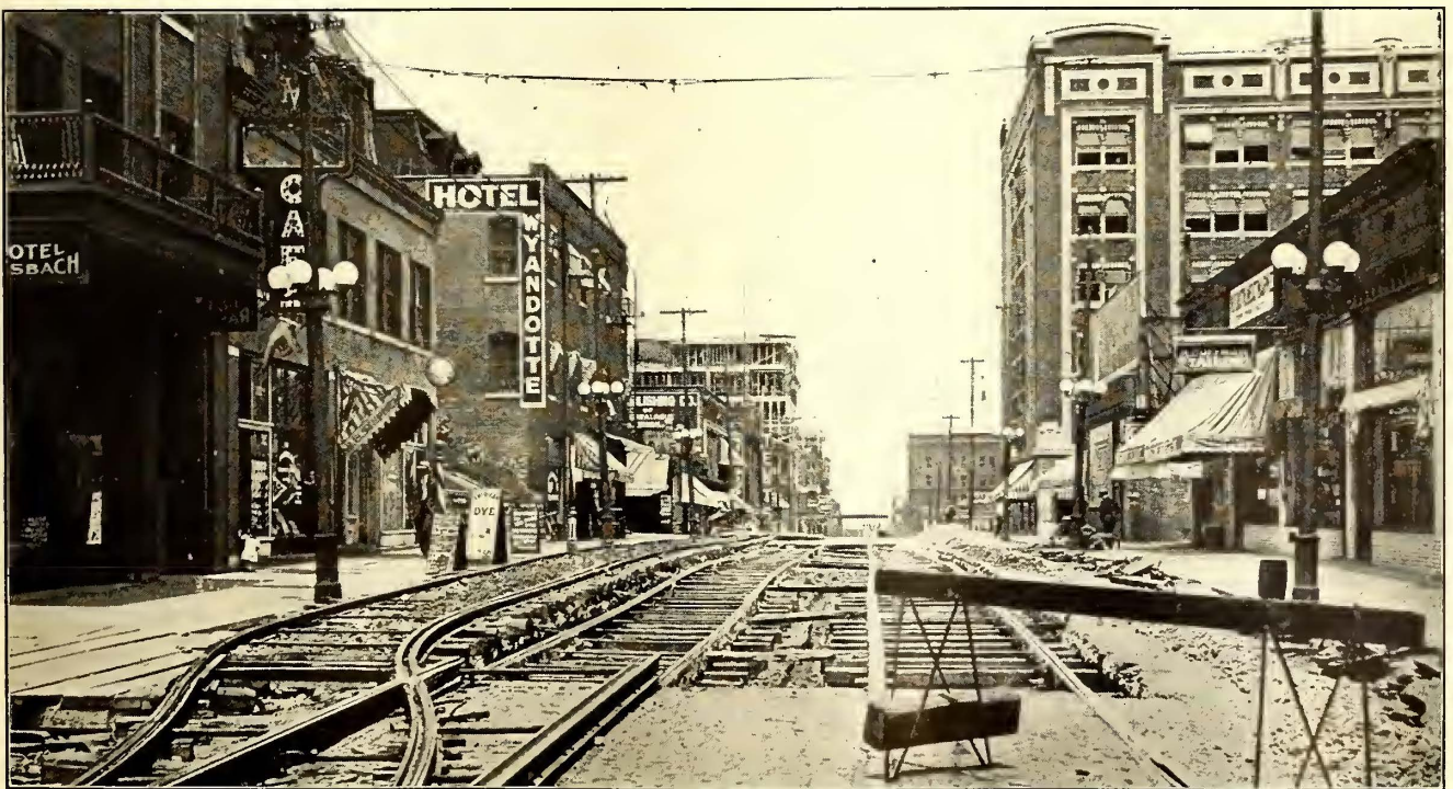
KANSAS CITY TRACK CONSTRUCTION—TEMPORARY TRACKS ON ABANDONED STREET
