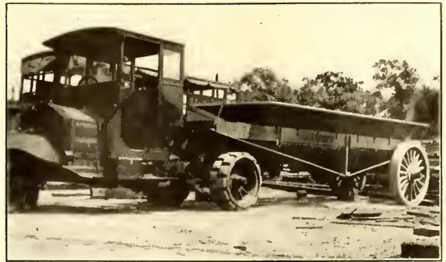
KANSAS CITY TRACK CONSTRUCTION—TRACTOR WITH STEEL DUMP BODY
