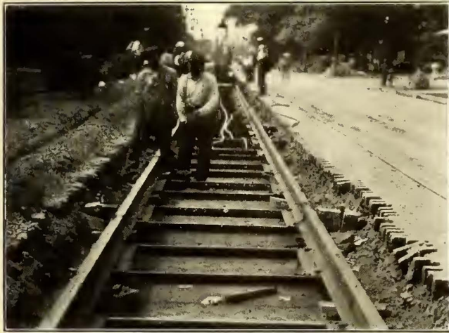
WORKMEN LEVELING TRACK IN AKRON, OHIO
