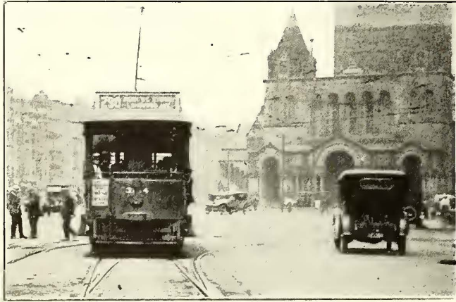
SOLENOID-OPERATED TRACK SWITCHES AT COPLEY SQUARE, BOSTON, MASS.
