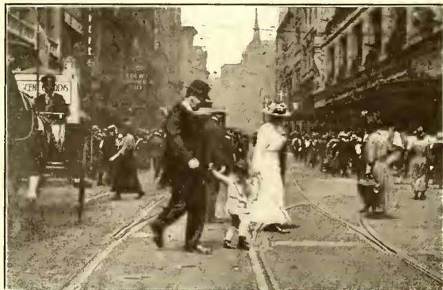
MOTOR-OPERATED TRACK SWITCHES AT THE BUSIEST CORNER IN NEW ENGLAND
