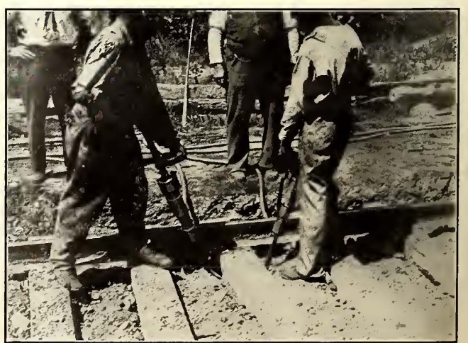
Pneumatic Tie Tamping—Figs. 9 and 10—Tamping Dirt-Gravel Ballast, on Lines of Indianapolis Traction & Terminal Company—Six Men with Shovels Replaced by Two Men with Machines
