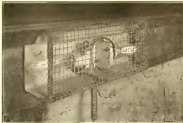
PIT LIGHTS IN SHOPS OF LEHIGH VALLEY TRANSIT COMPANY
