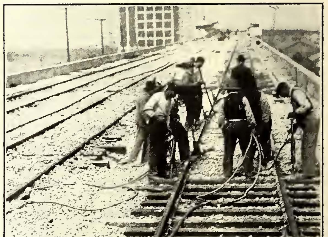
Pneumatic Tie Tamping—Fig. 8—Tamping Stone Ballast on Dual System of Rapid Transit in Queens Borough, New York City
