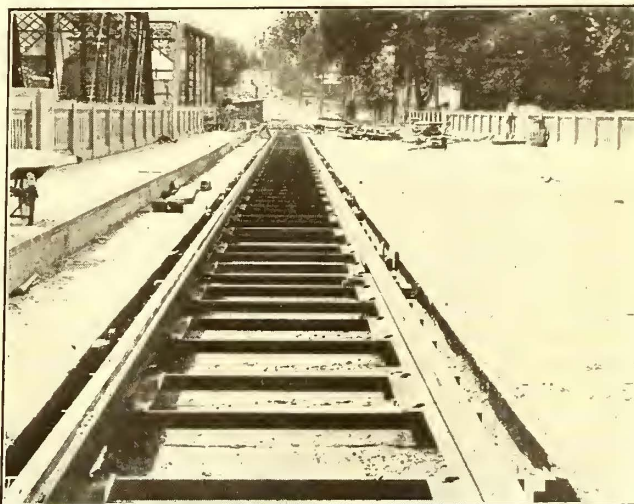
TRACK INSTALLATION ON CONCRETE BRIDGE, WARREN, OHIO
