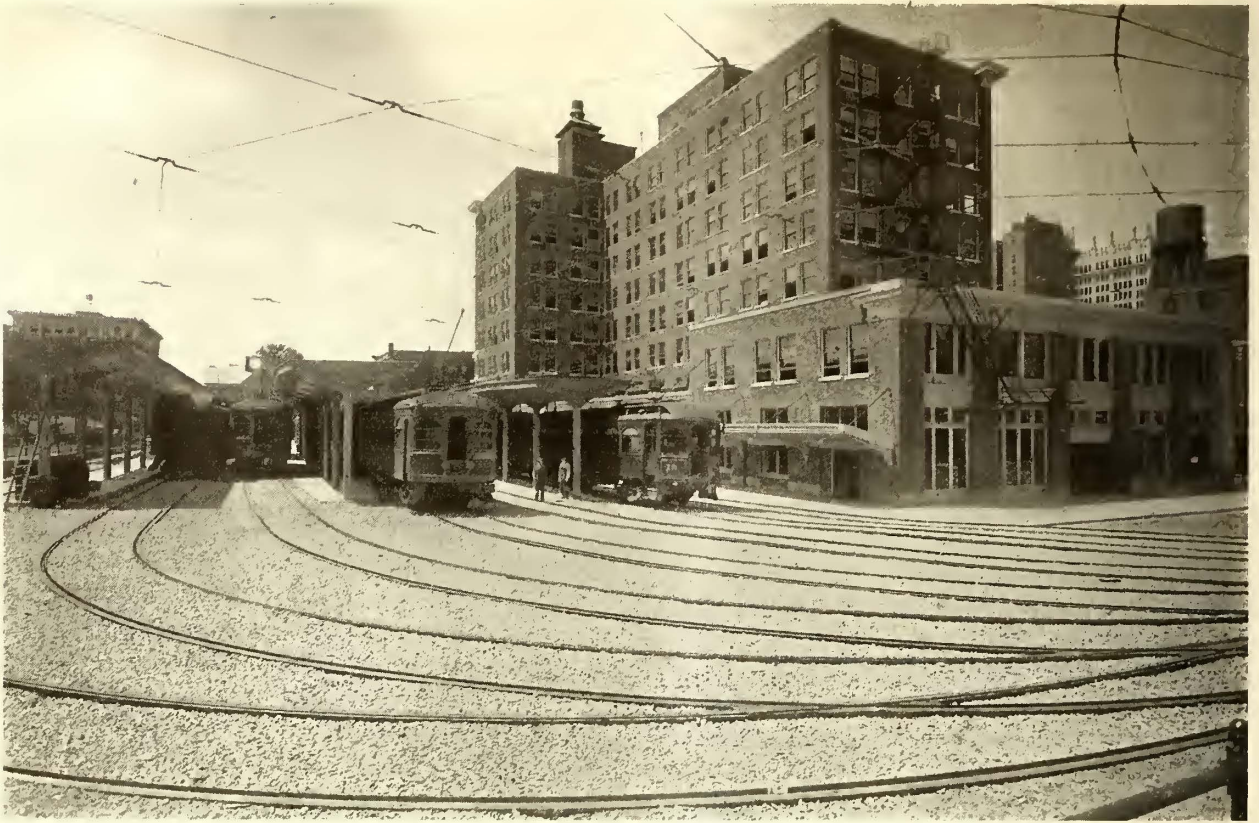
SEVEN THROUGH TRACKS SWINGING INTO TERMINAL YARD. VIEW TAKEN FROM POSITION A ON TRACK LAYOUT
