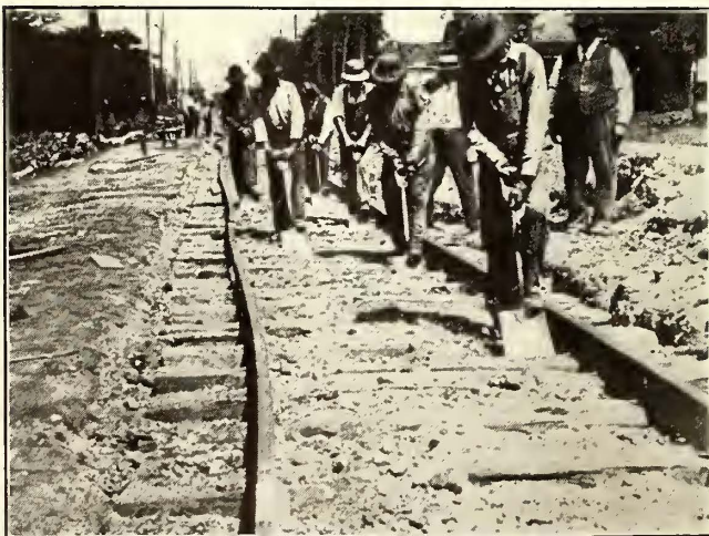
Pneumatic Tie Tamping—Figs. 9 and 10—Tamping Dirt-Gravel Ballast, on Lines of Indianapolis Traction & Terminal Company—Six Men with Shovels Replaced by Two Men with Machines
