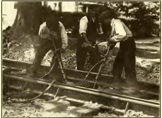
PNEUMATIC TIE TAMPING—FIG. 2—A WORKING UNIT. TWO MEN WITH TAMPERS AND ONE MAN SHOVELING BALLAST
