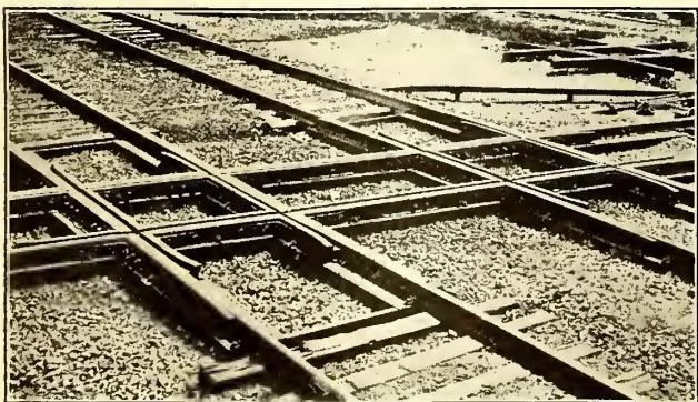
WOOD-BLOCK FILLED CROSSING, WELLINGTON, OHIO
