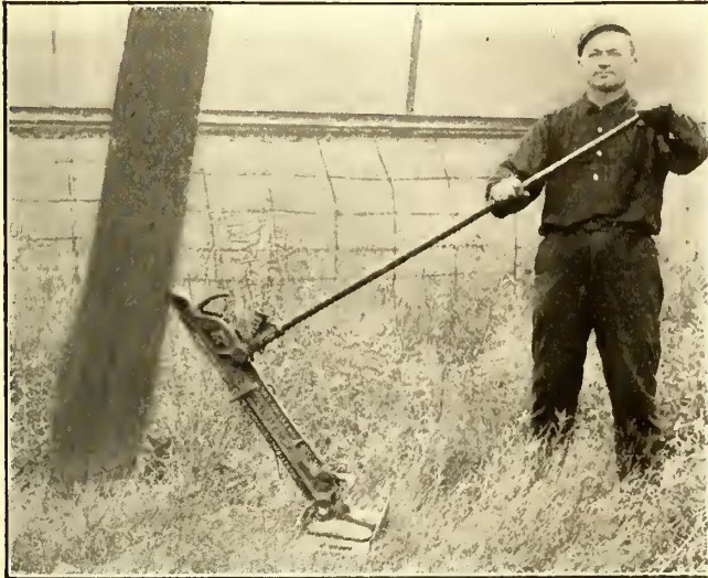
VIEW OF JACK IN POSITION FOR STRAIGHTENING POLE
