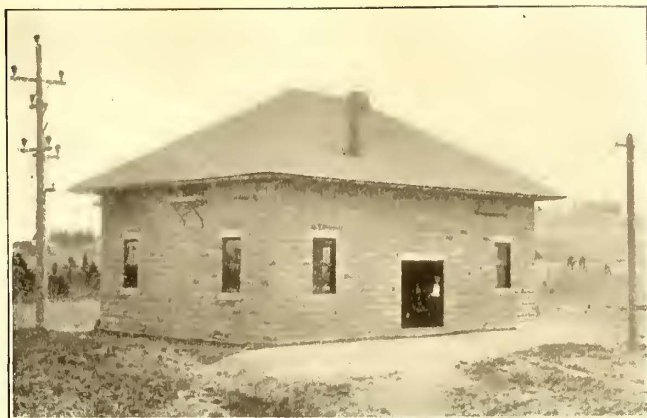
AROOSTOOK VALLEY RAILROAD—SUBSTATION AT CARIBOU
