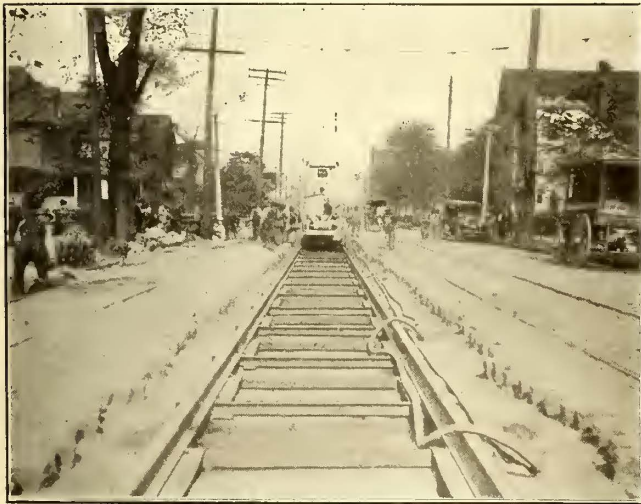
VIEW ON BROADWAY, SHOWING TEMPORARY TRACK AND CONCRETING GANG AT WORK
