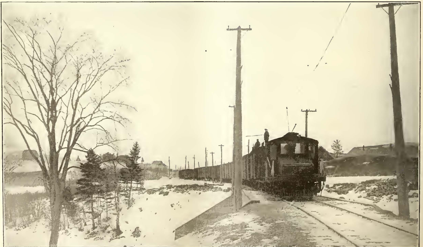
AROOSTOOK VALLEY RAILROAD—FREIGHT TRAIN HAULED BY 40-TON 1200-VOLT ELECTRIC LOCOMOTIVE
