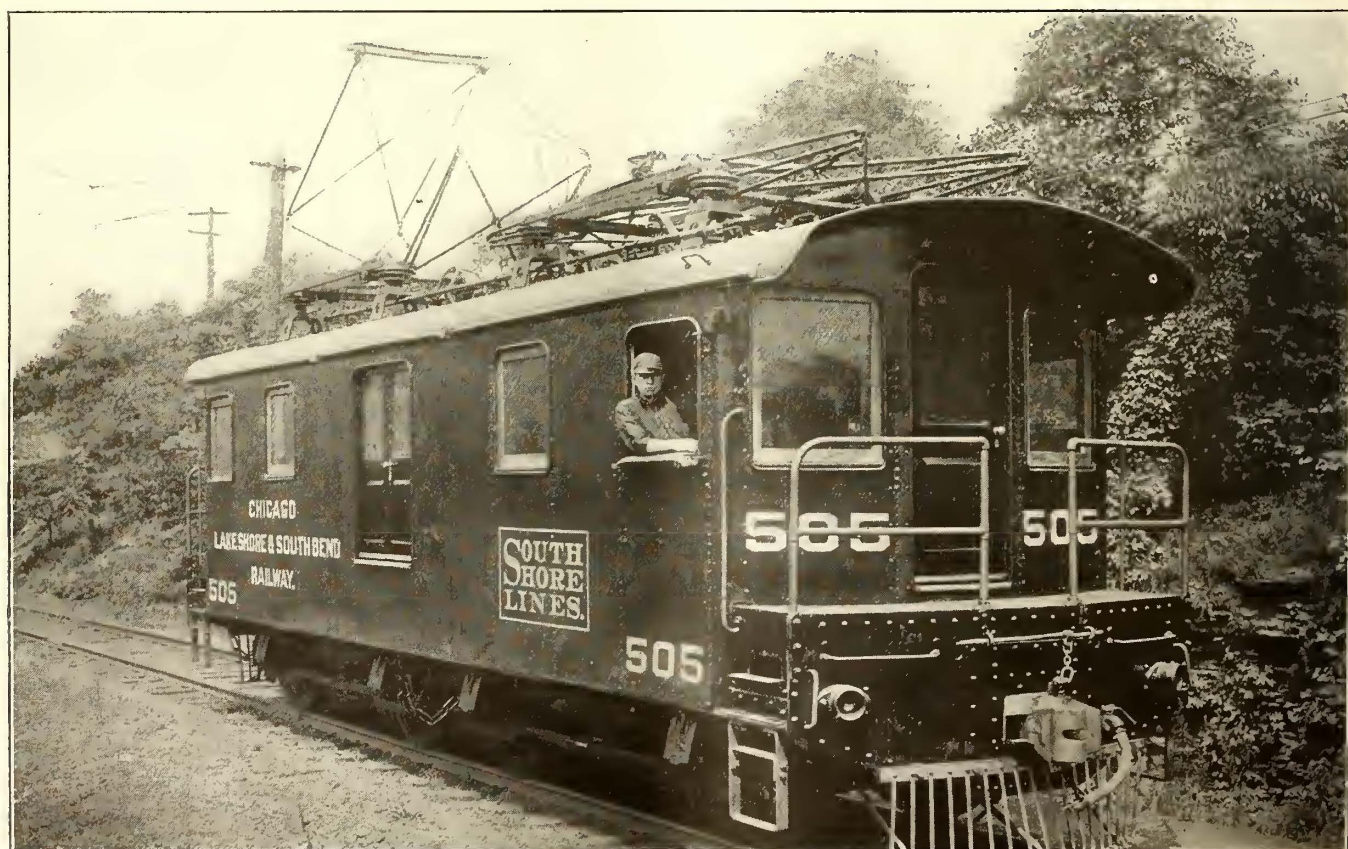
SOUTH SHORE LOCOMOTIVES—VIEW OF LOCOMOTIVE SHOWING BOX CAB WITH SIDE DOORS
