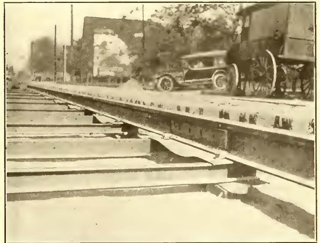
VIEW OF NEW TRACK BLOCKED UP READY FOR CONCRETING
