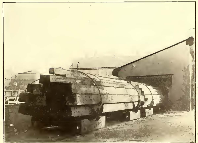
FIG. 8—CHARGE OF TIMBER READY FOR RETORT
