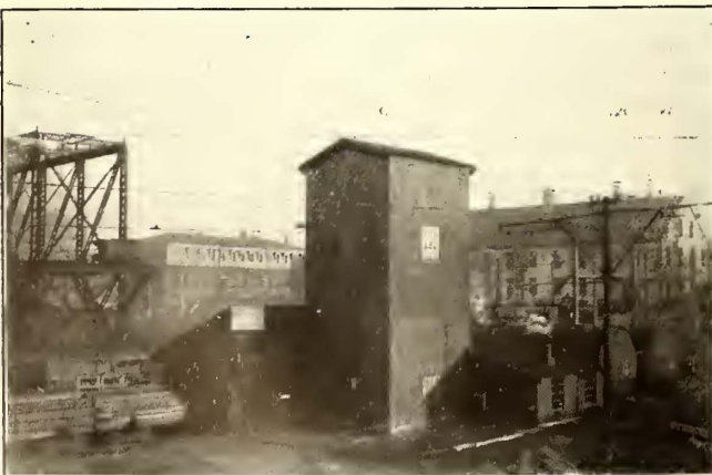
FIG. 3—GENERAL VIEW OF PLANT
