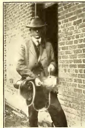
PORTABLE LAMPS IN USE BY TUNNEL INSPECTOR
