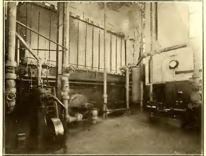
HOLYOKE POWER PLANT—FUEL ECONOMIZER, RESERVE BOILER FEED PUMP AND OTHER BOILER ROOM AUXILIARIES
