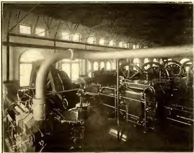
HOLYOKE POWER PLANT—ENGINE ROOM IN RECONSTRUCTED PLANT
