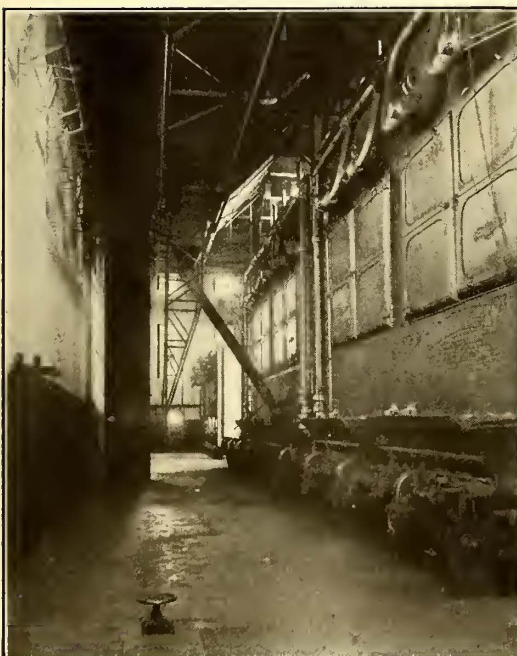
HOLYOKE POWER PLANT—FIRING AISLE IN BOILER ROOM; STOKERS, WITH ONE OF THE DUPLICATE STOKER ENGINES AND ONE OF THE DUPLICATE STEAM TURBINE BLOWERS FOR FORCED-DRAFT SYSTEM
