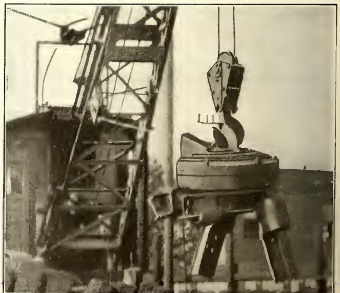
STORAGE YARDS—FIG. 19—ELECTROMAGNET USED BY CINCINNATI TRACTION COMPANY, LIFTING SCRAP MATERIAL
