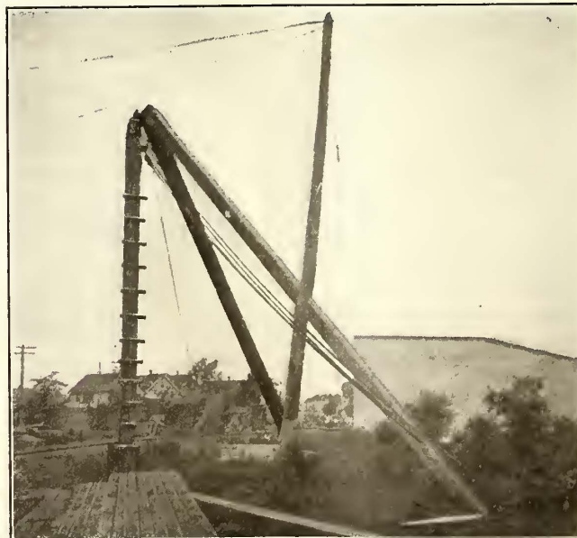
STORAGE YARDS—FIG. 2—STIFF-LEG DERRICK IN STORAGE YARD OF CONNECTICUT COMPANY, BRIDGEPORT, CONN.
