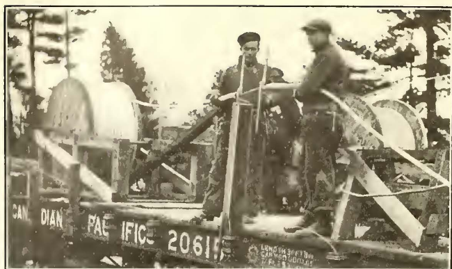
JOINING STEEL CORE WITH SPLICING SLEEVE
