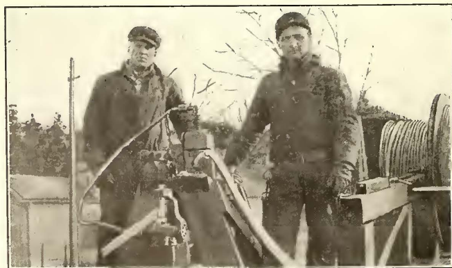
HYDRAULIC PRESS FOR JOINING ALUMINUM STRANDS IN SLEEVE
