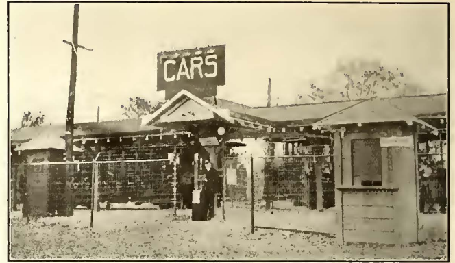
HANDLING FAIR TRAFFIC—LOADING PLATFORM AS SEEN FROM OUTSIDE AT SPRINGFIELD (MASS.) FAIR GROUNDS
