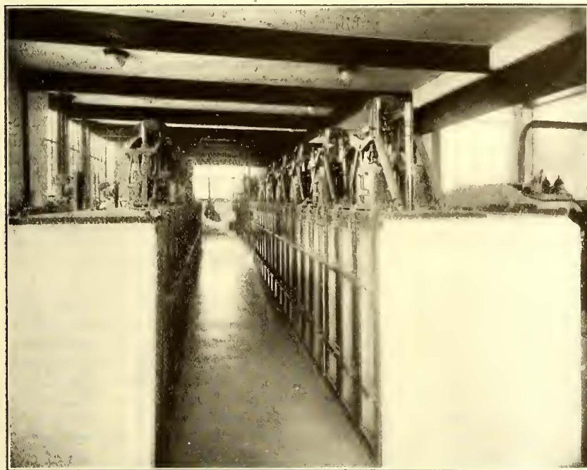
FREMONT POWER STATION—OIL SWITCHES ON TURBINE FLOOR; VIEW OF OIL-SWITCH COMPARTMENT
