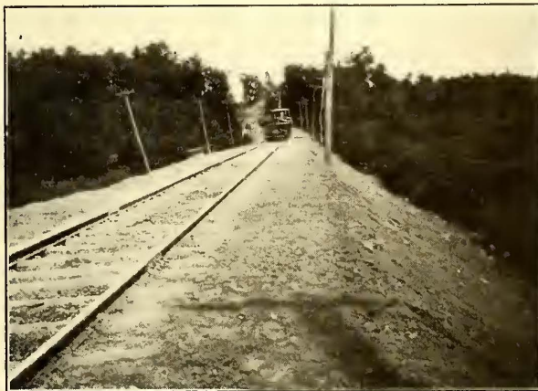
New Fill for Electric Railway Track
