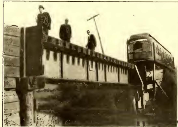
Electric Railway Bridge Structure
