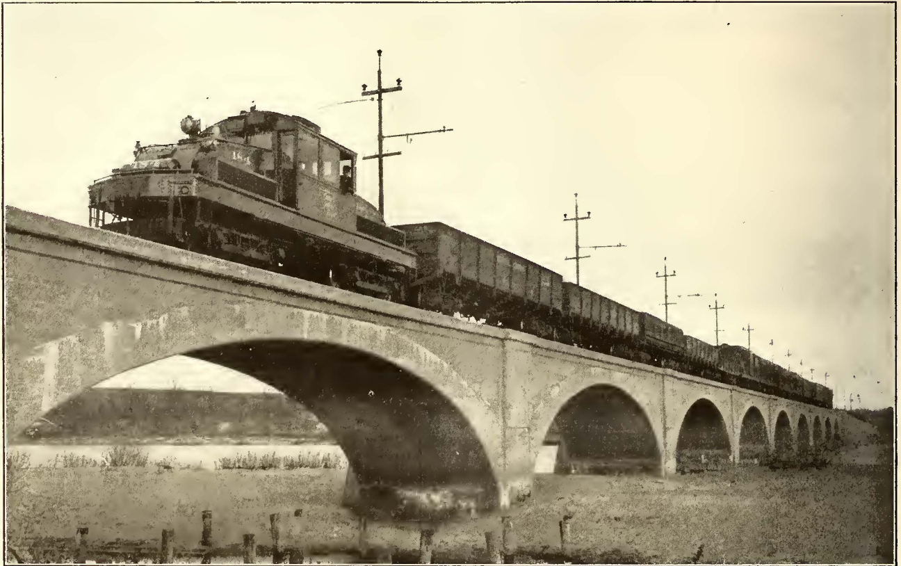
MILLER TROLLEY SHOE TRANSMITTING CURRENT FOR FREIGHT TRAIN ON WATERLOO, CEDAR FALLS & NORTHERN RY.
