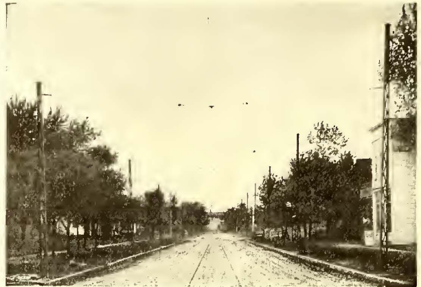
Bates Steel Poles in use by the DES MOINES CITY RAILWAY , Des Moines, Iowa, U. S. A.
