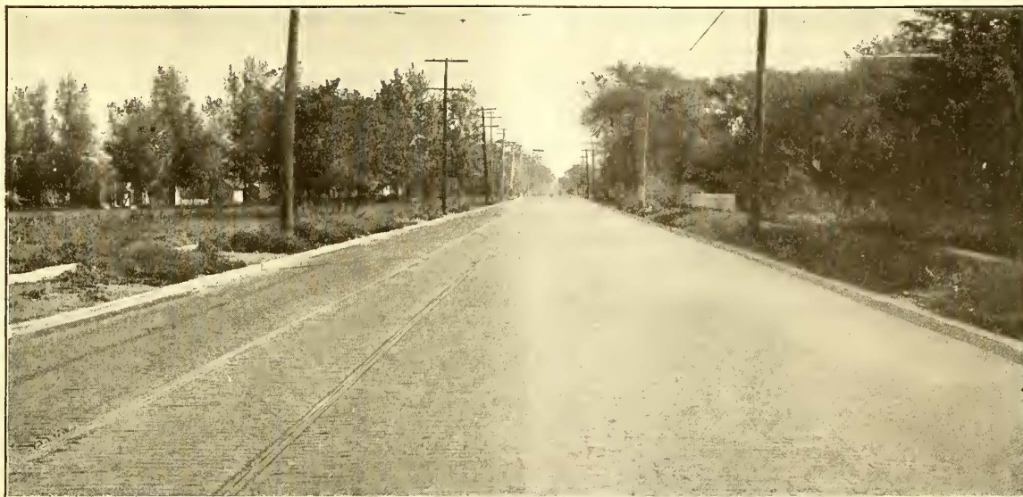
Rockingham Road, Davenport, Iowa. Brick pavement filled with Barrett's Paving Pitch.
