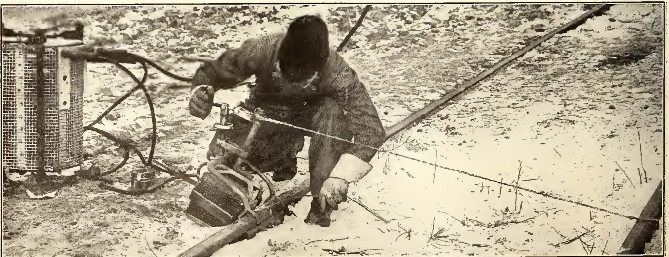
PORTABLE ELECTRIC WELDER IN USE UNMOUNTED
