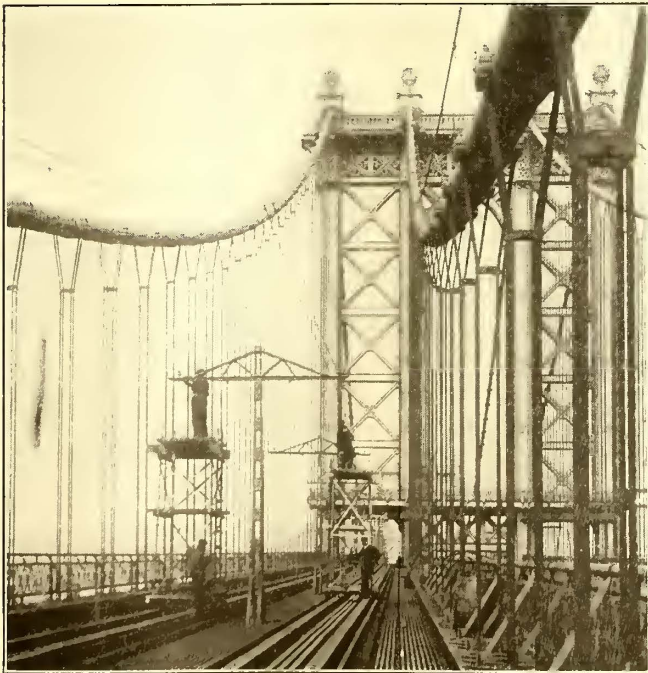
CATENARY TROLLEY CONSTRUCTION ON MANHATTAN BRIDGE—CONSTRUCTION GANGS ATTACHING HANGERS BETWEEN MESSENGER WIRE AND TROLLEY WIRE
