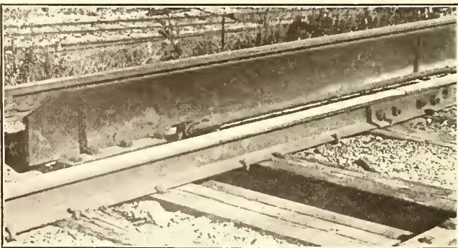
THIRD-RAIL PROTECTED BY BOARD AT THE SIDE
