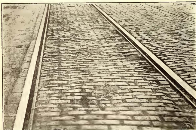
TRACK MAINTENANCE DATA—FIG. 7, SLAG BRICK PAVING SHOWING DAMAGE NOT CAUSED BY RAILWAY
