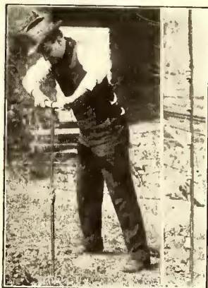
PREPARING TO BLAST A POLE HOLE; VIEW OF DYNAMITE STICK
