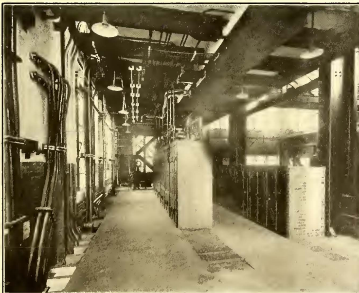
CONNECTICUT COMPANY POWER PLANT—OIL SWITCH AND BUSBAR COMPARTMENTS ON MIDDLE GALLERY—ALTERNATING-CURRENT AND DIRECT-CURRENT OPERATING PANELS ON TOP GALLERY IN TURBINE ROOM
