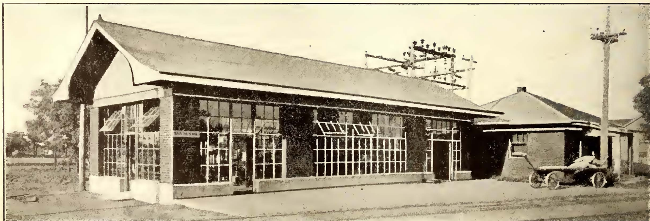
NEW KANSAS INTERURBAN—BURTON DAYLIGHT SUBSTATION
