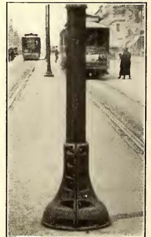
CAST-IRON SLEEVES TO PROTECT AND REINFORCE CENTER TROLLEY POLES AT GROUND LINE
