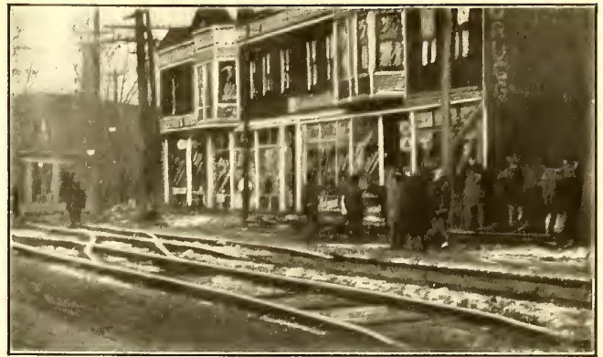
VIEW OF PORTION OF TEMPORARY TRACK WORK
