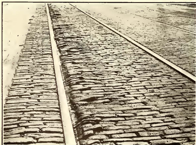
UNEVEN PAVING ALONG OUTER RAIL DUE TO ATTEMPT TO HAVE TRACK GRADE FOLLOW CROWN OF STREET
