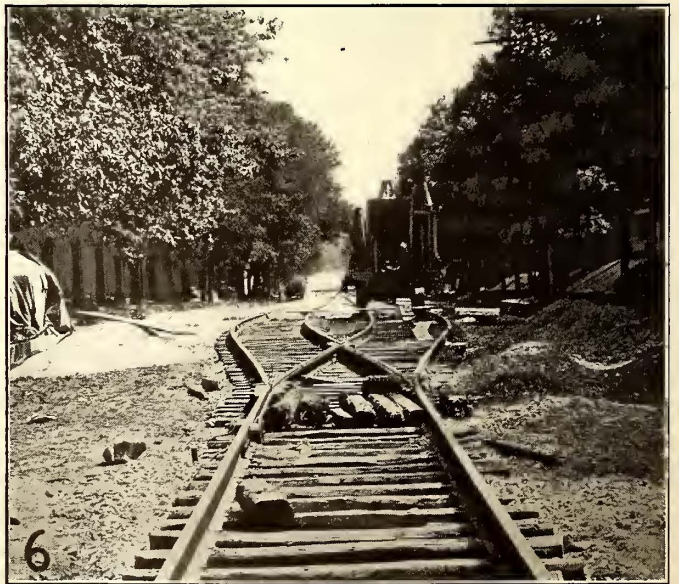
for granite nose blocks. Fig. 5.—Double track reduced to single track at intersection to save space and cost. Fig. 6.—Residence track construction. Note temporary flanges on traction wheels of concrete mixer.
