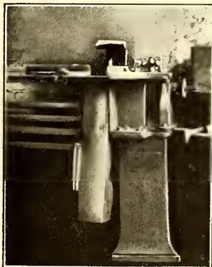
MACHINE FOR CUTTING CARBON BRUSHES
