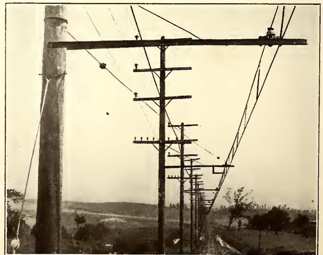
VIEWS ON SAN BERNARDINO LINE OF PACIFIC ELECTRIC RAILWAY SHOWING OVERHEAD CONSTRUCTION WITH STEEL CONTACT WIRE
