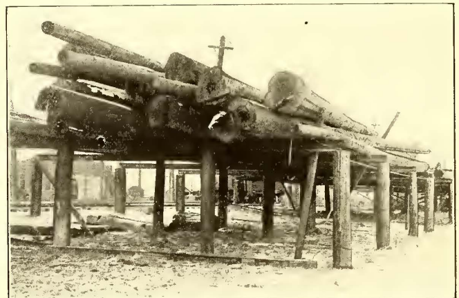
POLE STORAGE STRUCTURE ON AN OHIO ELECTRIC LINE
