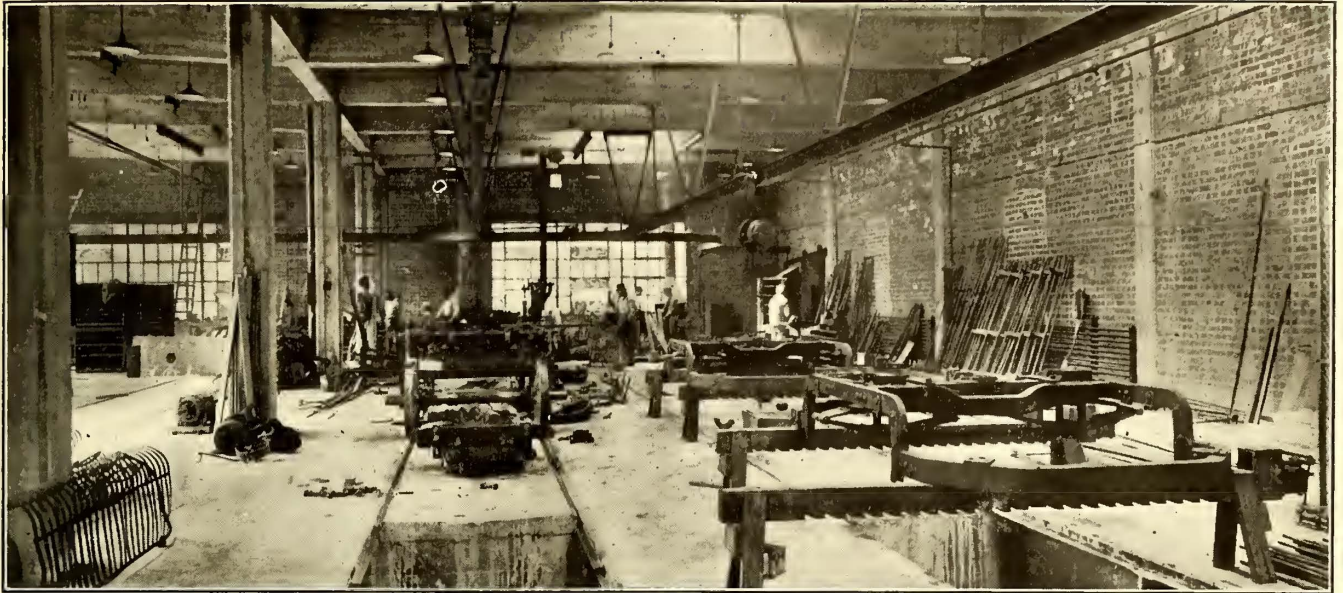
ROCK ISLAND SHOPS—TRUCK SHOP EQUIPPED WITH MONO-RAIL TRAVELING HOISTS
