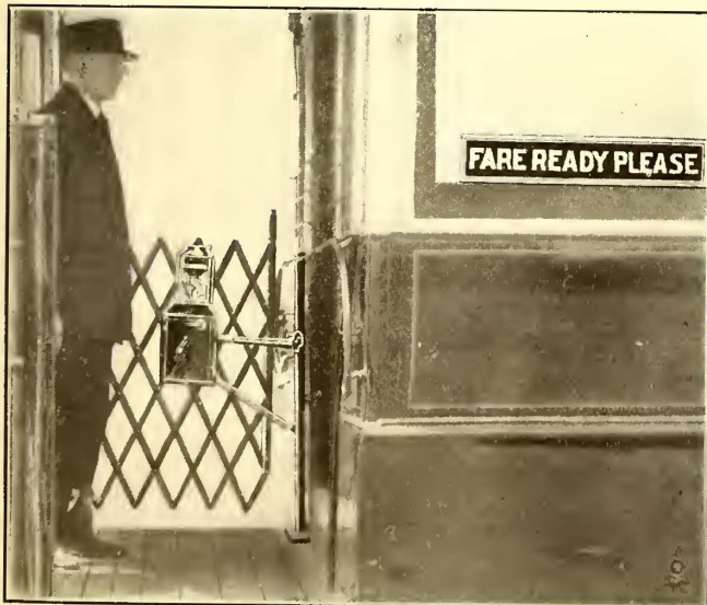
INEXPENSIVE FARE-BOX BRACKET AND PAPER WINDOW SIGN
