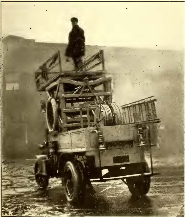
FIG. 5—TYPICAL LINE TRUCK OF CLEVELAND RAILWAY
