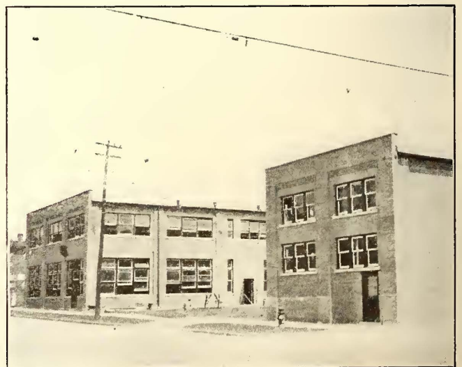
DETROIT FREIGHT TERMINAL—FRONT ENDS OF BUILDINGS HOUSING OFFICES
