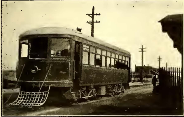
STORAGE-BATTERY CAR BEING CHARGED AT POINT SHIRLEY, MASS.
