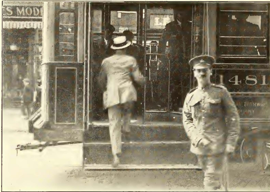
MONTREAL DOOR EQUIPMENT—VIEW OF REAR PLATFORM ON REMODELED CAR
