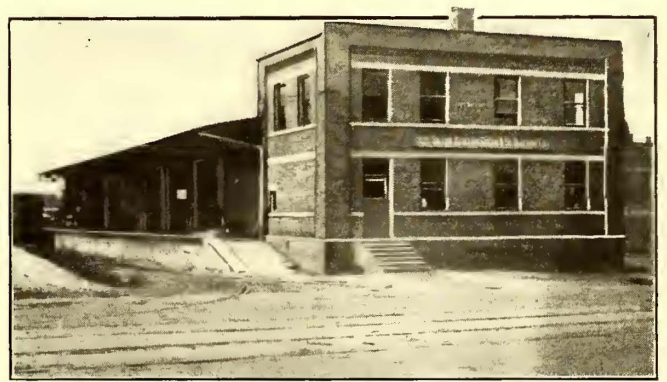
T., B. G. & S. T. CO.—FREIGHT TERMINAL AT TOLEDO, SHOWING AUTOMOBILE LOADING PLATFORM
