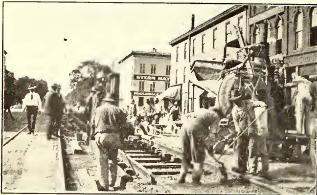
POURING CONCRETE AROUND DAYTON MECHANICAL TIES
